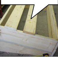
The upper part is made of 2x4, 2 boards of 6 feet long and 4 boards of 3'1" wide
